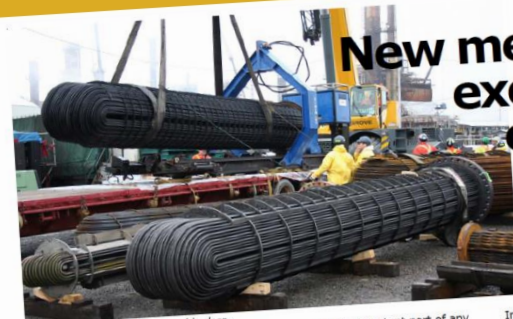
The exchanger in the foreground is clean, the one in the background is ready for its bath.
